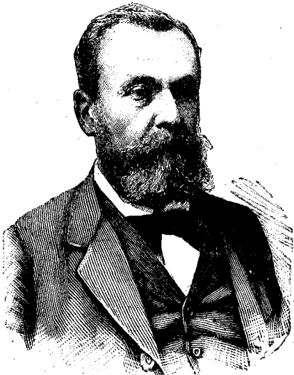
M. MARUÉJOULS (Travaux publics)
